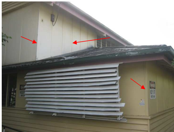
Photograph 15: External: Main Hall building ; East side (level 1) – Wall battens and corner guards
