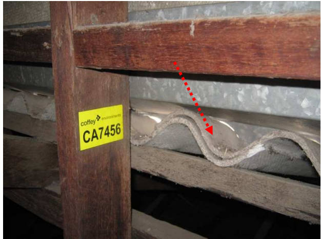
Photograph 3: Internal: Level 1, South side Stage – Fire stairs; Above ceiling lining. Asbestos cement fragments (wall lining) and asbestos ceiling lining.
