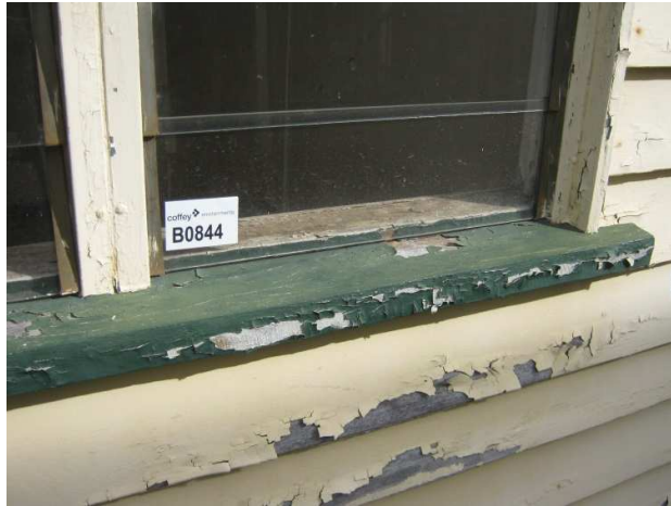
Photograph 23: External: Main Hall building; Ground level, north side windows – Timber frame rail (horizontal): Lead-based paint, Refer to paint sample BO844
