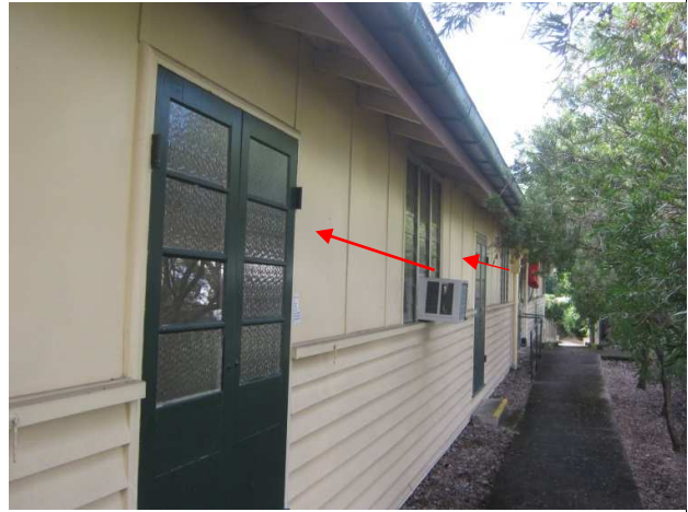
Photograph 14: External: Main Hall building ; South side (level 1) – Asbestos cement wall cladding sheets
