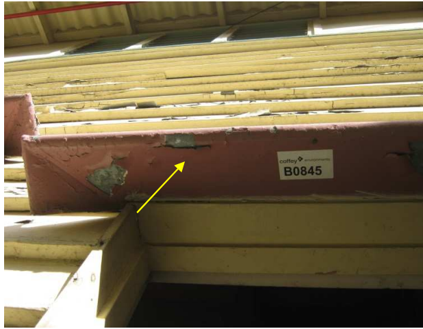
Photograph 25: External: Main Hall building; Ground level, north side windows – Metal window shades. Lead-based paint
