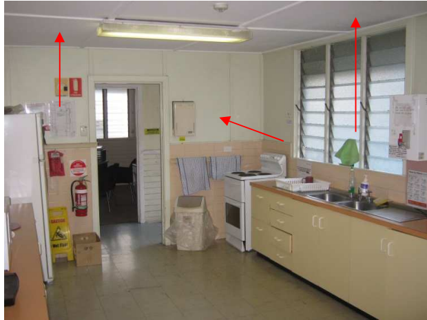
Photograph 11: Internal: Level 1, North side Caretakers accommodation – Kitchen; Asbestos cement ceiling and wall lining.
