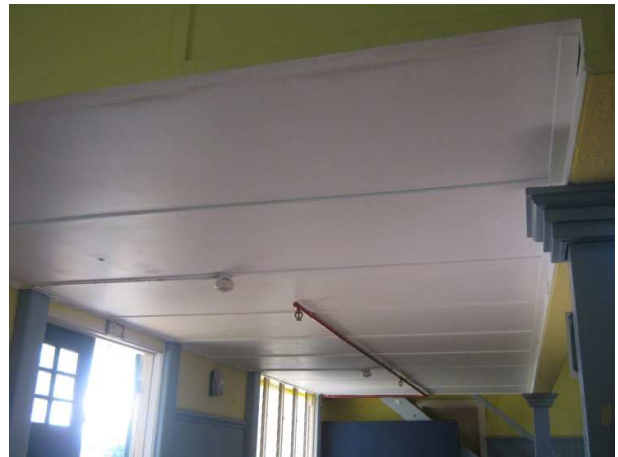
Photograph 8: Internal: Level 1, Mezzanine Cinema room – Under-croft ceiling lining. Asbestos cement sheets.
