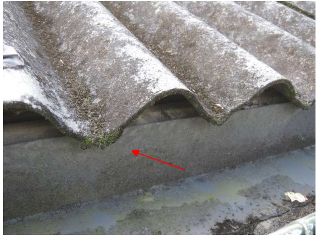
Photograph 19: Accommodation building, Ground level sub-floor area – Below north west side stairs; Asbestos cement fragments. Refer to sample CA7478
