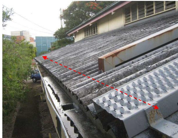
Photograph 16: External: Main Hall building, Level 1 ; South side lower roof – Roof cladding sheets; Corrugated asbestos cement. Refer to sample CA 7474
