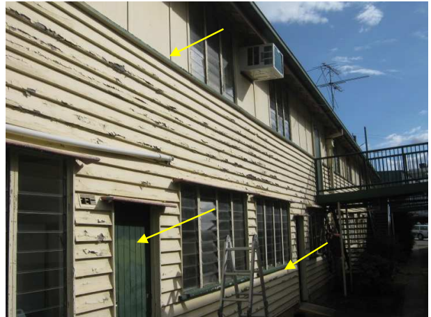
Photograph 24: External: Main Hall building; Ground level, north side windows – Timber frame rail (horizontal); and doors (x2), Lead-based paint system
