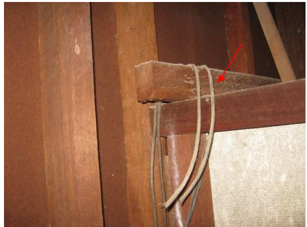
Photograph 4: Internal: Level 1, North side Stage area – Rostrum; Hanging wiring with suspected asbestos cloth insulation.
