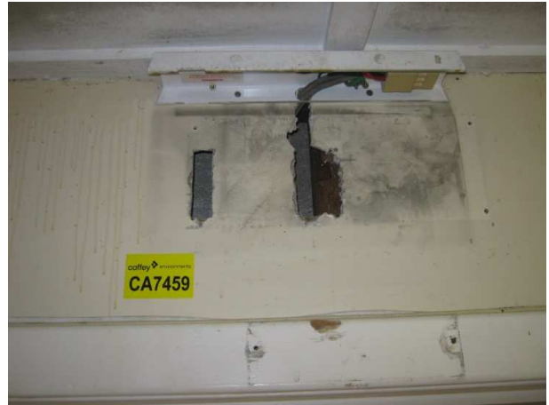
Photograph 6: Internal: Level 1, South side First Aid / Meeting room – South wall lining (Midway). Damaged asbestos cement lining. (former EXIT sign)
