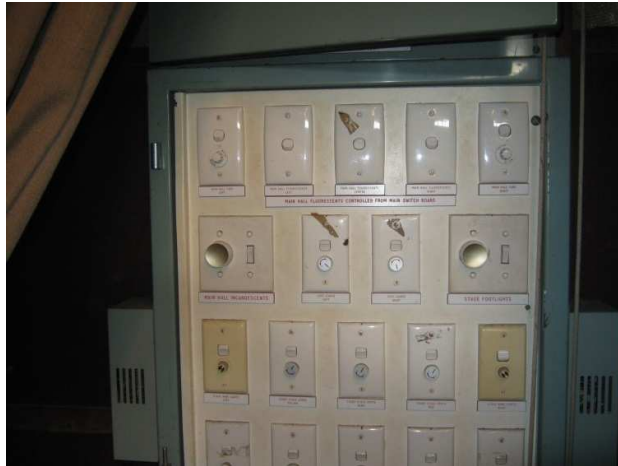
Photograph 5: Internal: Level 1, South side Stage area – Main Switchboard and D.B; Suspect 'Zelemite' E.M.B support.
