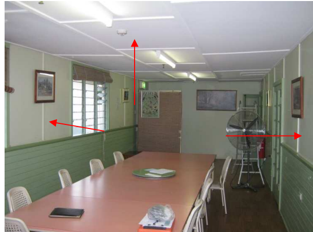
Photograph 10: Internal: Level 1, North side Red Cross Dining / staff room – Ceiling and wall lining. Asbestos cement sheeting. Please refer to samples CA 7462 and CA 7460
