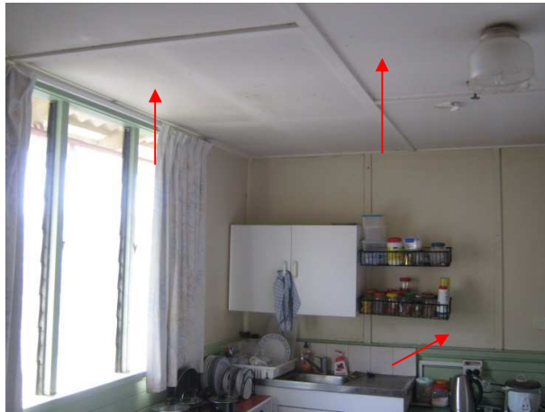
Photograph 11: Internal: Level 1, North side Caretakers accommodation – Kitchen; Asbestos cement ceiling and wall lining.
