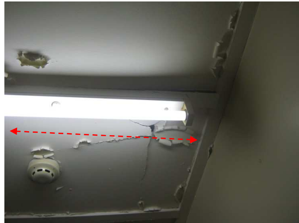
Photograph 12: Internal: Level 1, North side Caretakers accommodation (supervisor) – Storage closet; Damaged ceiling sheet.
