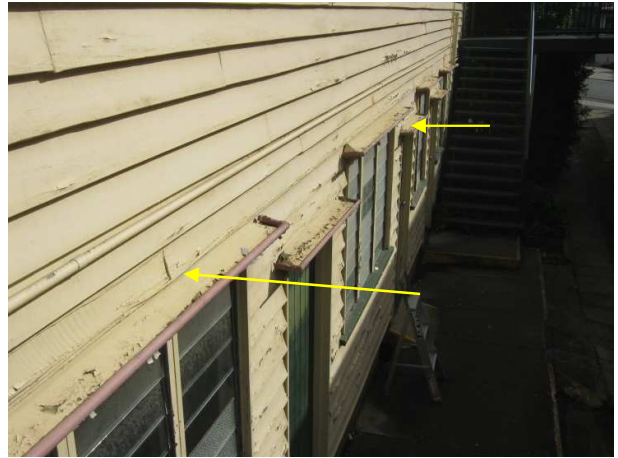
Photograph 26: External: Main Hall building; Ground level, north side windows and doors – Metal window shades. Refer to paint sample B0845, Lead-based paint.
