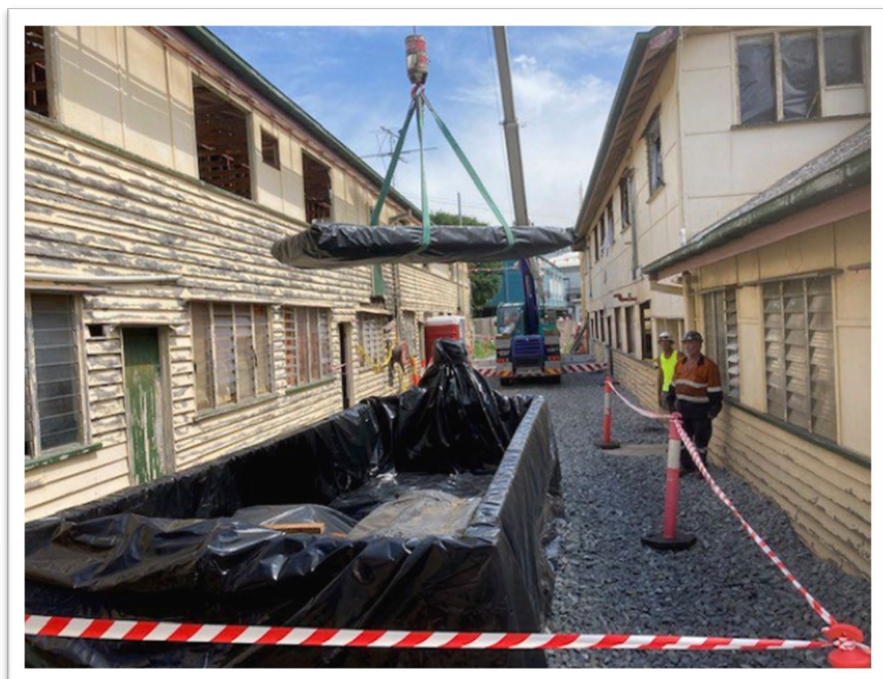
Figure 22. DOUBLE-WRAPPED PACKS BEING CRANED DOWN INTO LINED ASBESTOS WASTE SKIP.
