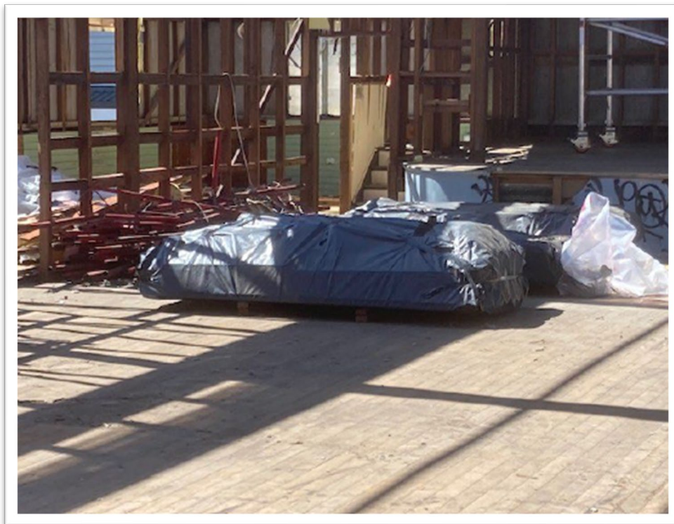
Figure 26. HANDLING AND ENCAPSULATION OF ACM SHEETING.
