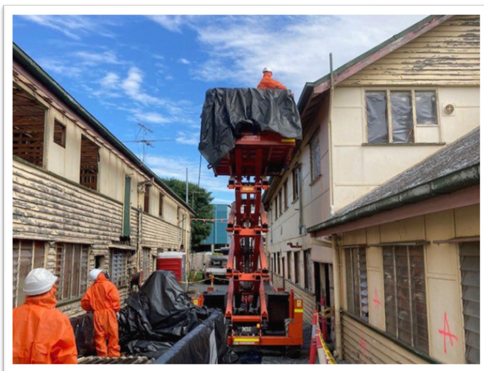
Figure 24. EWP (SCISSOR LIFT) BEING USED TO LOWER ACM SHEETING FOR TRANSFER TO WASTE SKIP
