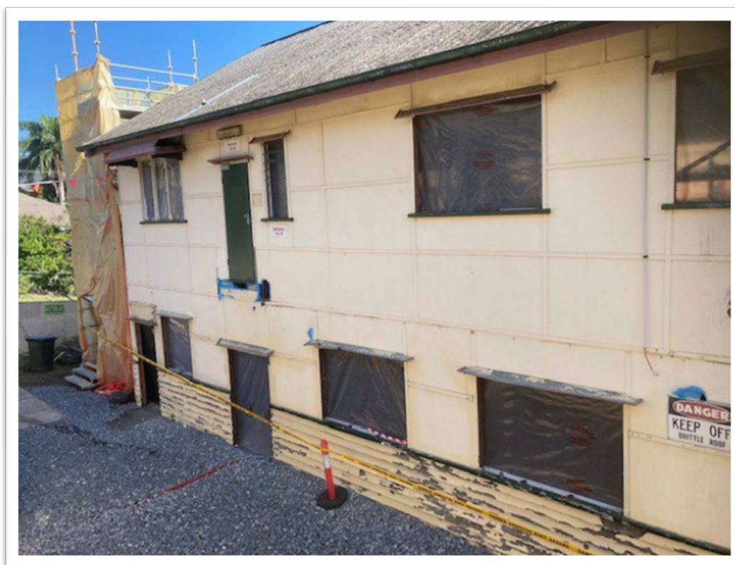
Figure 9. ACCOMMODATION BLOCK WITH BOTH LEVELS ENCAPSULATED WITH 200UM RATED PLASTIC TO ALL OPENINGS IN PREPARATION FOR BOTH FRIABLE AND NON-FRIABLE ASBESTOS REMOVAL.
