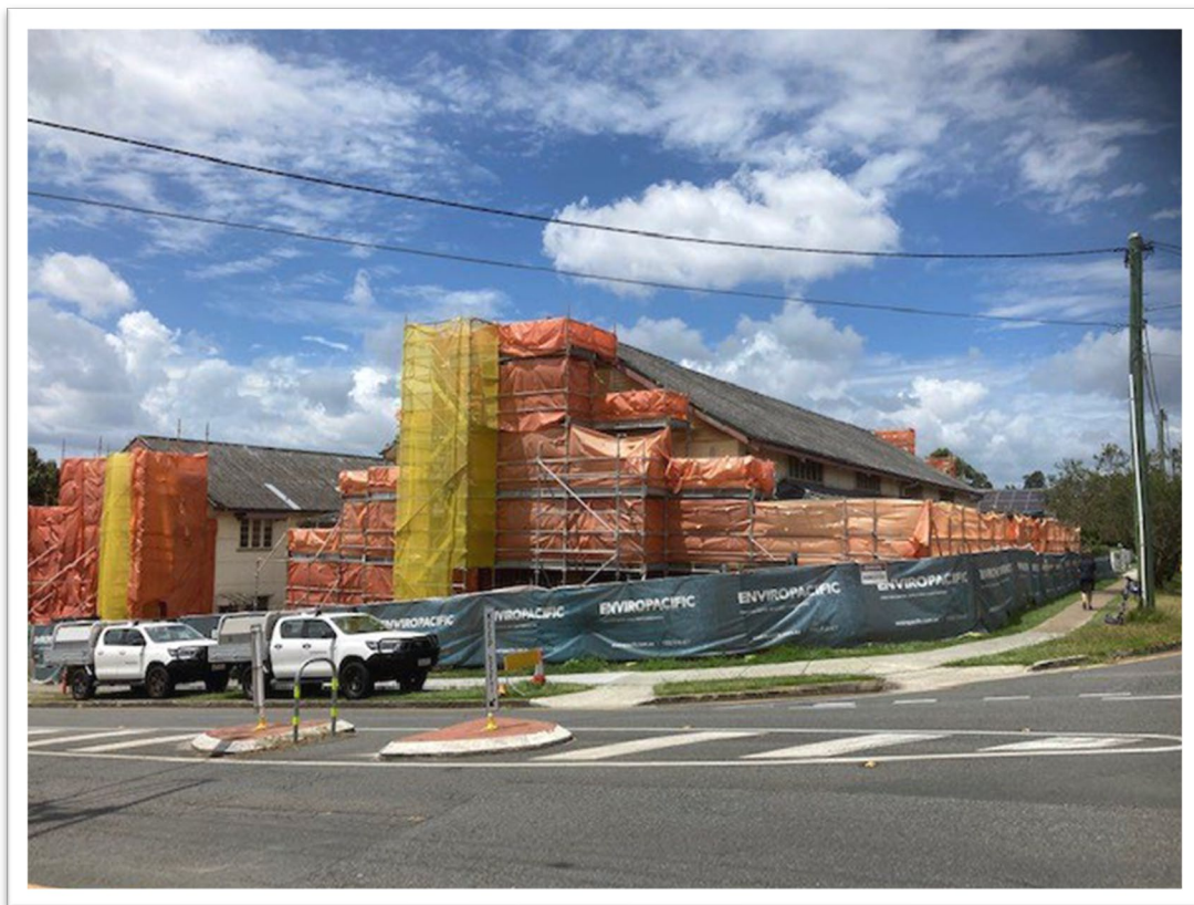
Figure 7. EXTERNAL SCAFFOLD WITH 200UM PLASTIC SHEET RE-INSTALLMENT TO PROVIDE A SEMI-ENCAPSULATION FOR THE NON-FRIABLE ASBESTOS REMOVAL WORKS
