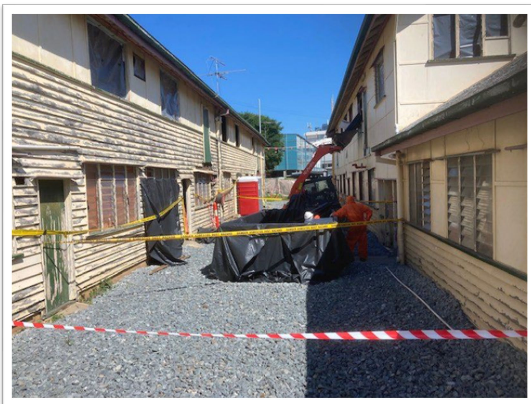
Figure 15. EXCLUSION ZONES / BARRIERS IN PLACE WHILE ENCAPSULATED BUNDLES OF THE ASBESTOS WASTE BEING LOWERED FROM UPPER LEVEL FOR MANUAL LOADING INTO THE DOUBLE LINED WASTE BIN.
