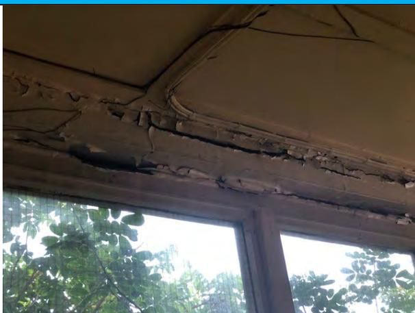
This image shows the existing damage to the section where the roof adjoins to the masonry front.
