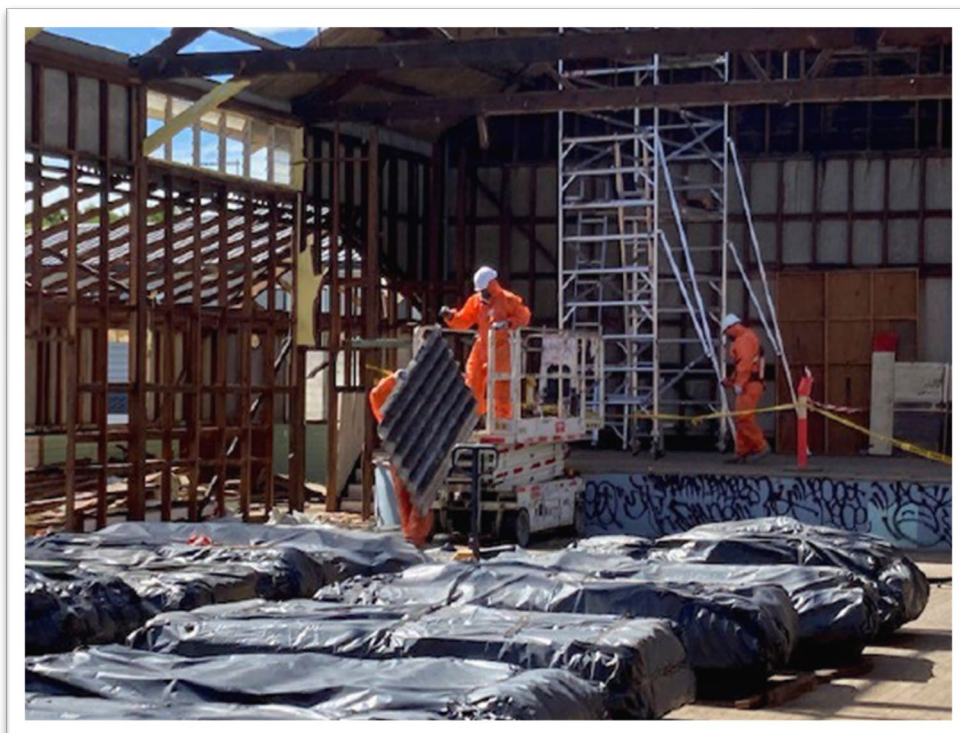
Figure 26. HANDLING AND ENCAPSULATION OF ACM SHEETING.
