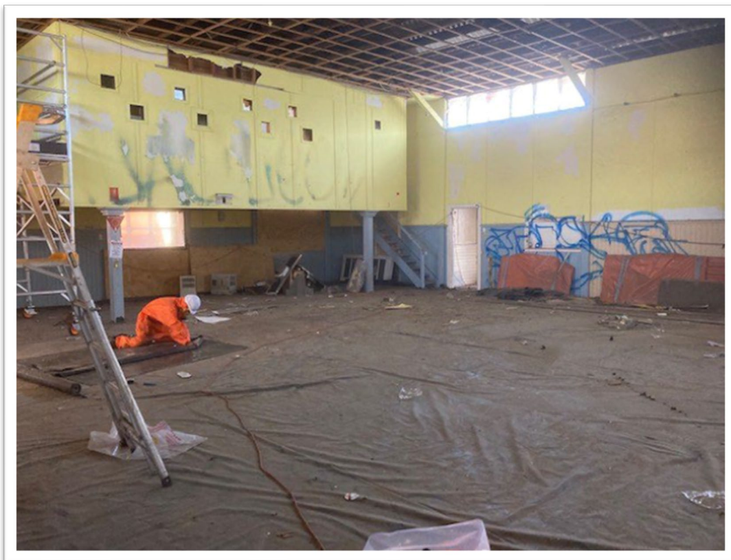
Figure 11. FRIABLE ASBESTOS REMOVAL
