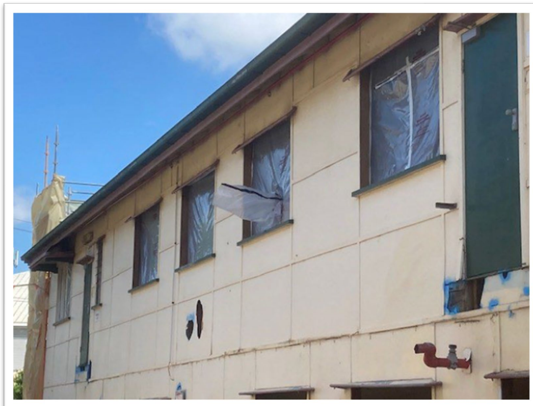
Figure 10. NEGATIVE AIR PRESSURE EXHAUST VENT HORIZONTAL, SHOWING NEGATIVE PRESSURE ENVIRONMENT BEING MAINTAINED FOR ASBESTOS REMOVAL WORK TO ENSURE CONTAINMENT OF ASBESTOS.
