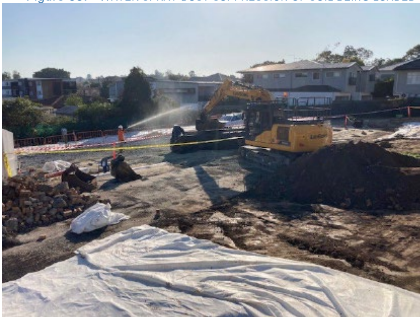
Figure 33. WATER SPRAY DUST SUPPRESSION OF SOIL BEING LOADED INTO SKIP
