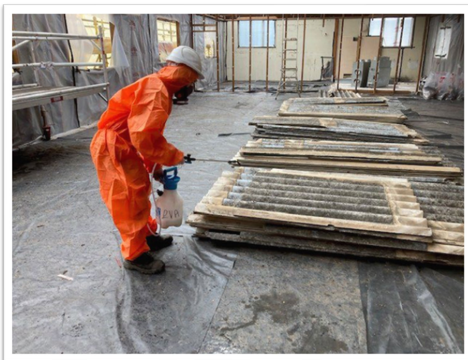
Figure 23. PVA SEALANT BEING APPLIED TO ACM SHEETING PRIOR TO HANDLING FOR LOAD OUT.
