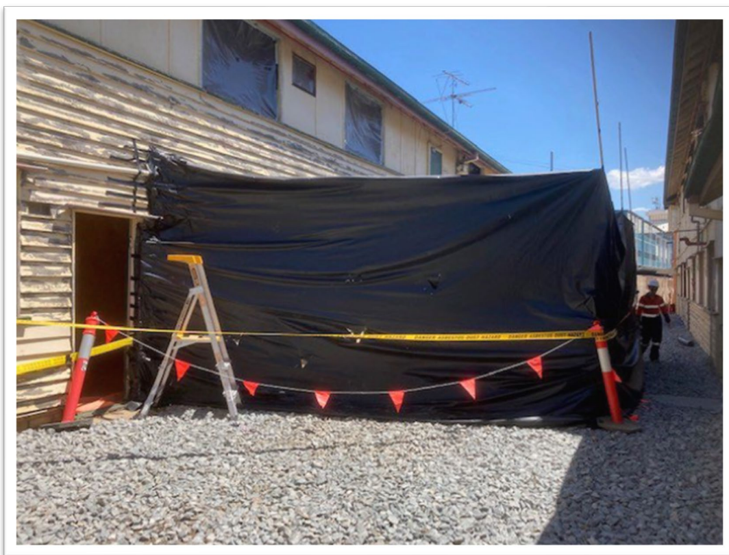
Figure 14. LOCALISED EXCLUSION ZONE FOR THE PURPOSE OF LOADING OUT ASBESTOS WASTE INTO LINED SKIP.
