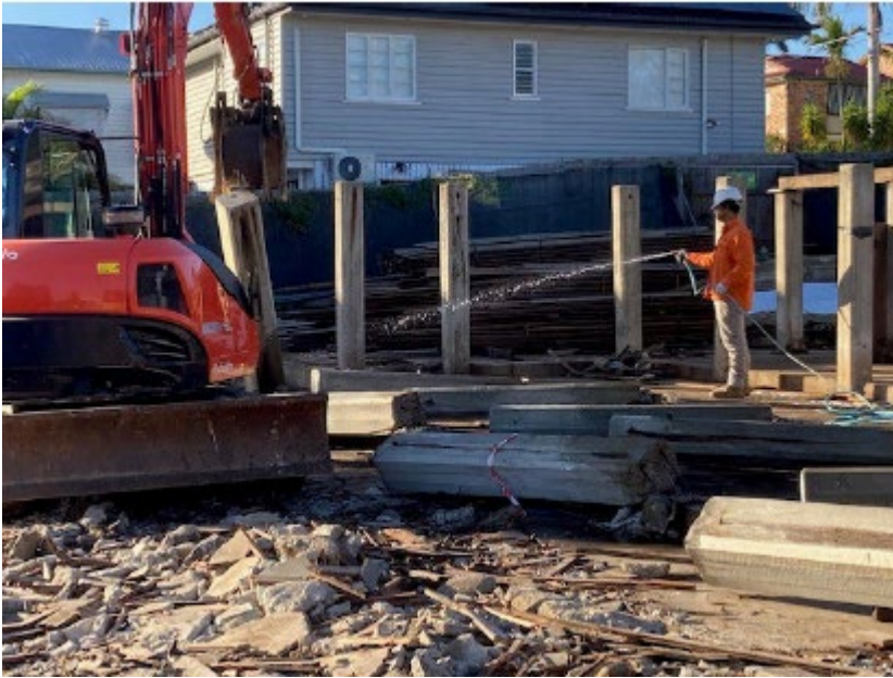
Figure 34. WATER SUPPRESSION DURING MECHANICAL DEMOLITION
