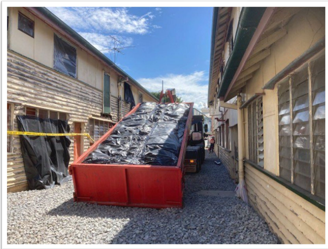
Figure 16. ASBESTOS WASTE LOAD OUT WITH BIN DOUBLE LINED AND AIRTIGHT.
