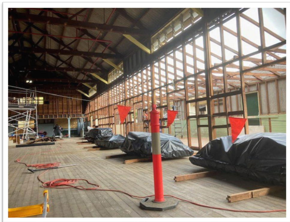
Figure 21. VARIOUS ENCAPSULATED PACKS READY FOR CRANING
