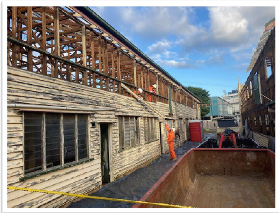
Figure 28. CONTROLLED REMOVAL OF THE EXTERNAL TIMBER (ACM PAINT)
