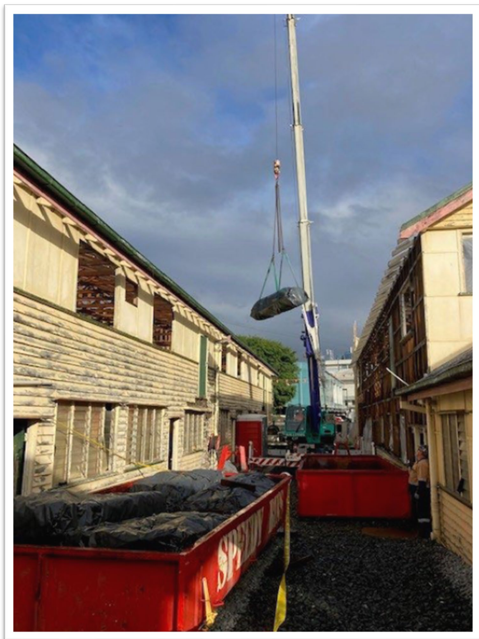
Figure 27. DOUBLE WRAPPED BUNDLES OF ASBESTOS WASTE BEING CRANED DOWN IN SOFT SLINGS
